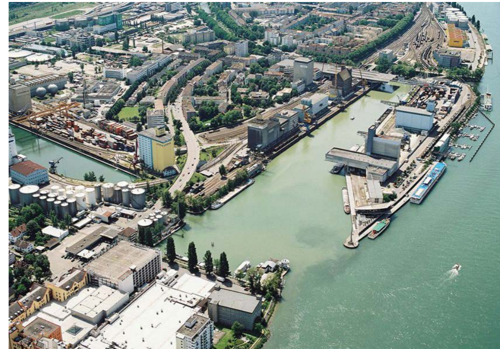
3Land project gathering Switzerland, Germany and France, the Basel Trinational Eurodistrict / © ETB
